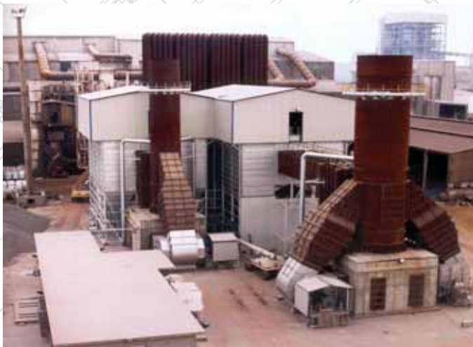
Fabripulse XLC serving an EAF and AOD in Spain Flow: 850,000 m 3 /h + 500,000 m 3 /h
