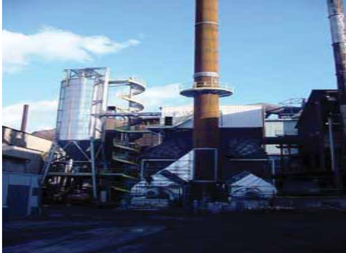
Fabripulse XLC serving an EAF in France Flow: 310,000 m 3 /h
