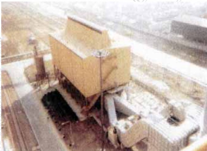
AMERtherm serving an EAF in China Flow: 1,600,000 m 3 /h
